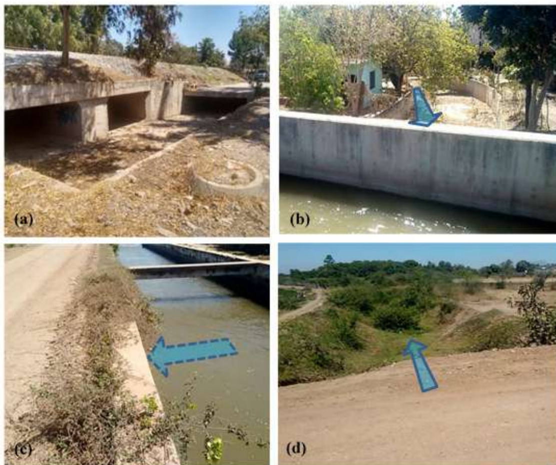
Figure 9. Evidence of changes in the drainage pattern due to agricultural and urban infrastructure. (a) Culvert drains runoff under a railroad. (b) Concrete-lined open ditch passes under a channel bridge. (c) Runoff drains to lateral channel. (d) Unlined ditch passing under a channel bridge.
